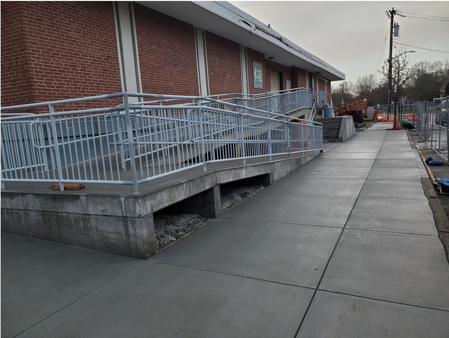
The new fully accessible main entrance to the Gath Pool bathhouse is substantially complete and we just poured the new sidewalks out front.
