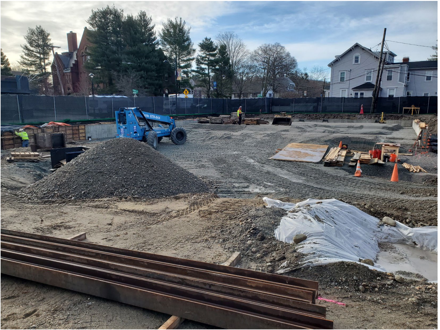
The bulk of the foundation has been poured now and the footprint of the building is starting to take shape.
