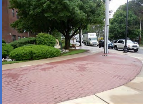
Stamped Concrete Walkway
