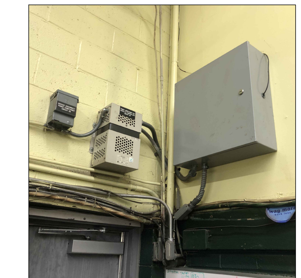
4 EXISTING IRRIGATION CONTROL CABINET E2.0
