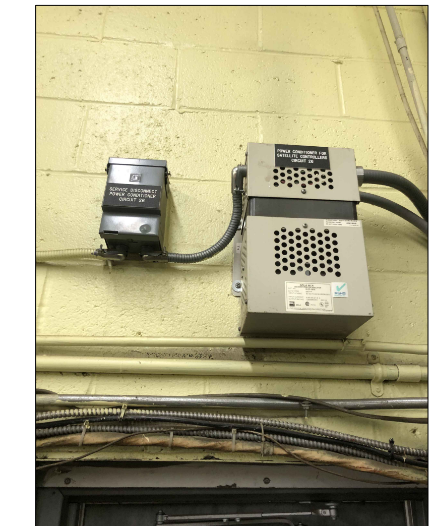
3 EXISTING IRRIGATION POWER CONDITIONER E2.0
