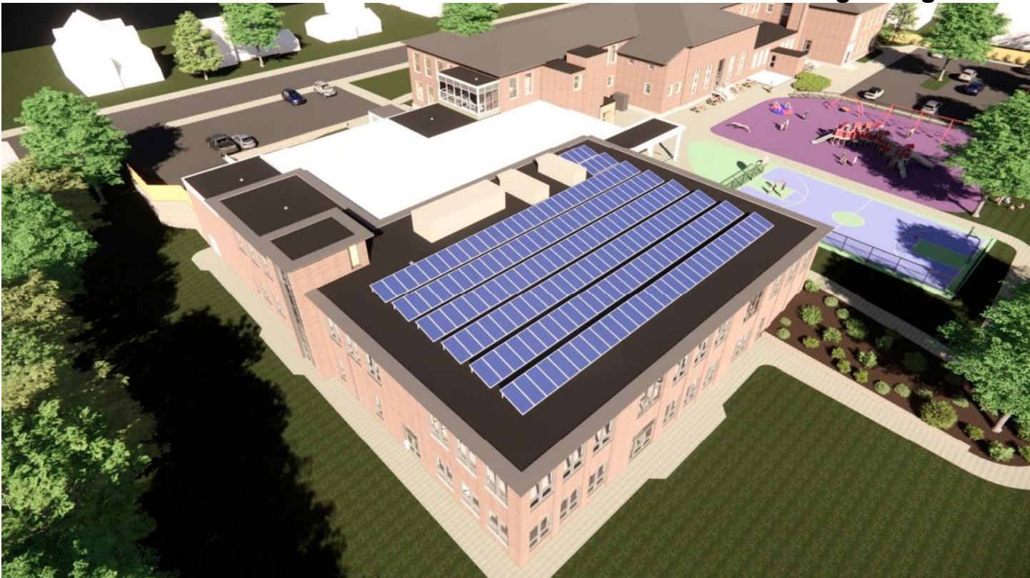
The above image shows the aerial view of the new addition with solar panels on the roof. In the upper righthand corner you can see the new playground and basketball court.
