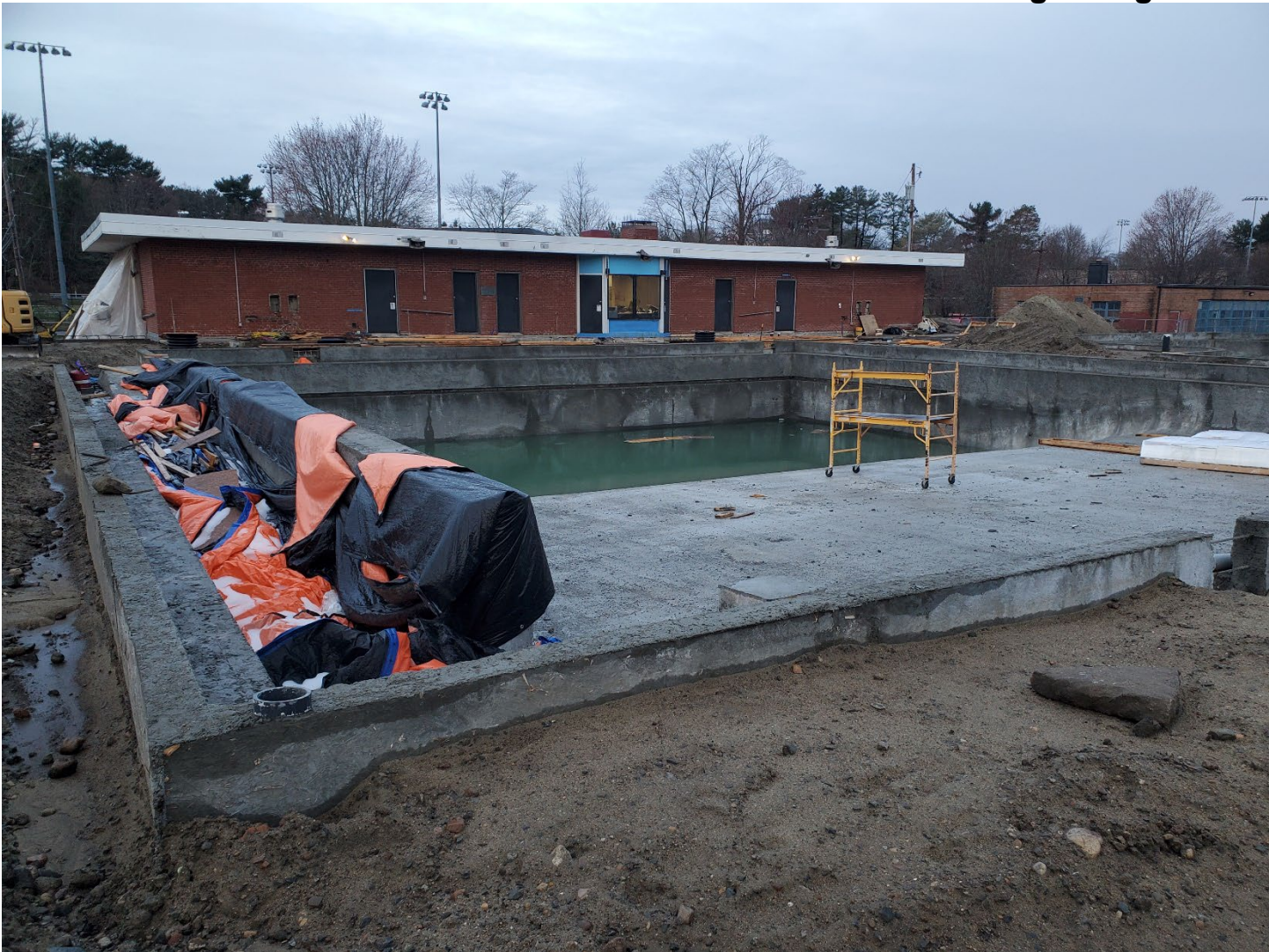
The two new pools are fully poured, and the new pool gutters are being installed. On the left you can see the ramp that will allow people of all abilities to enjoy the competition and lap pool. The splash pads will be located to the right of this image.
