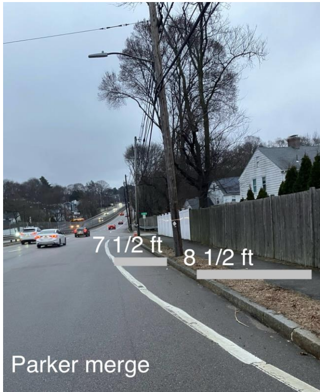
8.5' to 16' available for the Parker Rt 9 east ramp (breakdown lane starts at 0')
