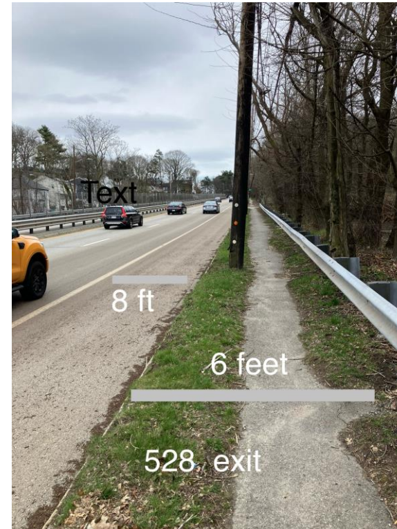
14 ft after exiting the project for vehicles and pedestrians, not 25'. Note the hill, requiring a longer merge.
