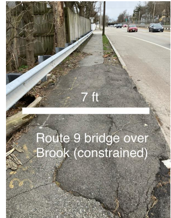
The bridge over Paul Brook, the abutters' fences and trees are all constraints to widening.
