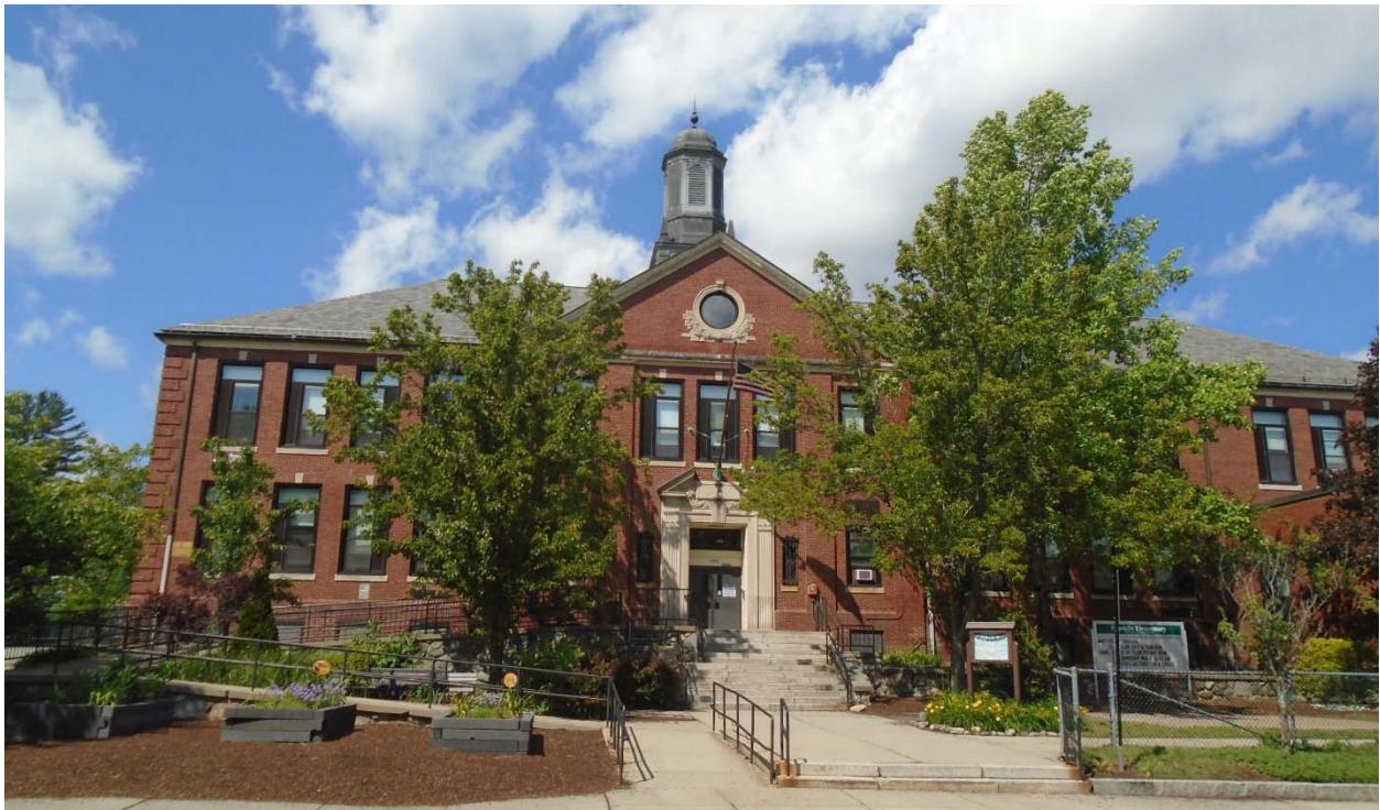
Existing Franklin Elementary School
