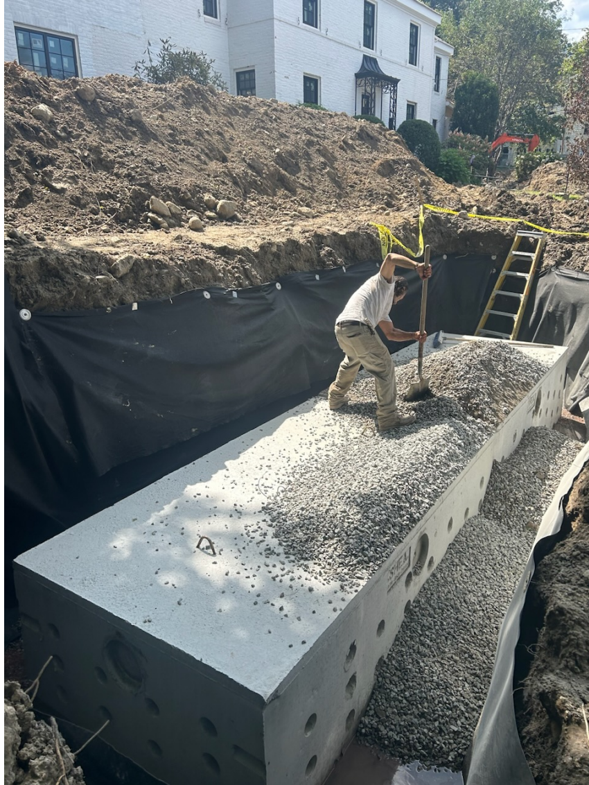
Precast leaching chambers being installed
