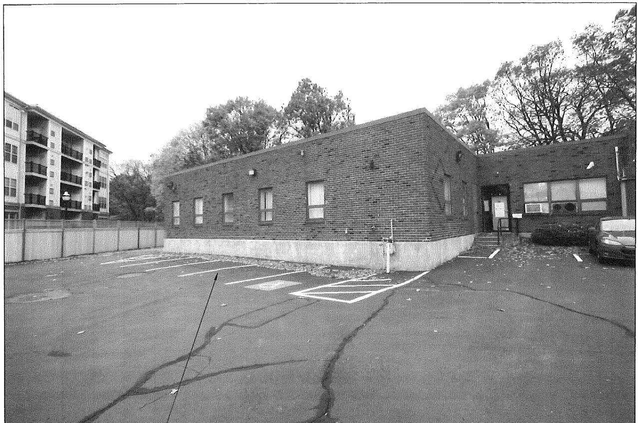
RELOCATE H-CAP AND ADD 1 NEW PARKING SPACE IN THIS AREA, SEE SKA-10
