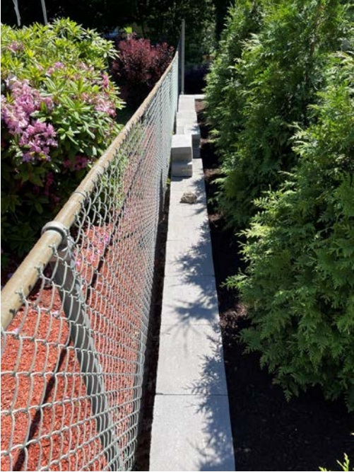
3. Rear Wall ~ extra blocks laying on top
