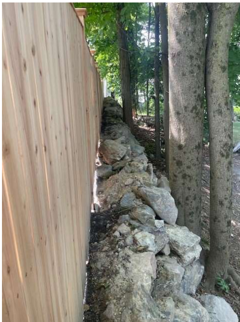
Rock Retaining Wall
