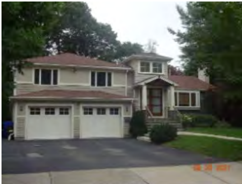
Sumner and Cynthia Victor House 81 Deborah Road (1955, altered) Source: Newton assessors' cards
