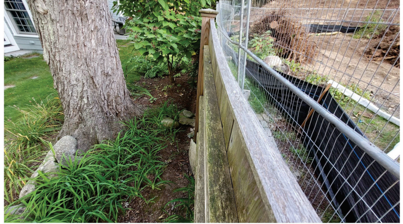
30 Woodhaven Rd (left), 56 Upland Rd (rt), Waban, (where developer plans to raise grade 2 ft)
