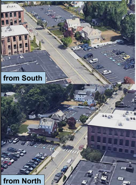
Google Earth View of 56 Chapel
