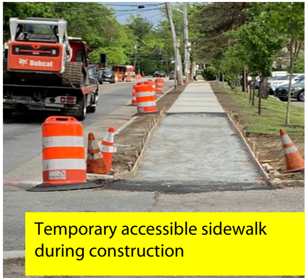
Temp. Asphalt ramp & temp cross walk painted
