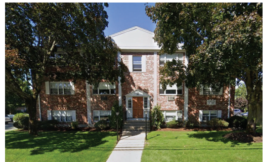
181 LEXINGTON STREET WITH BOILER ROOM
