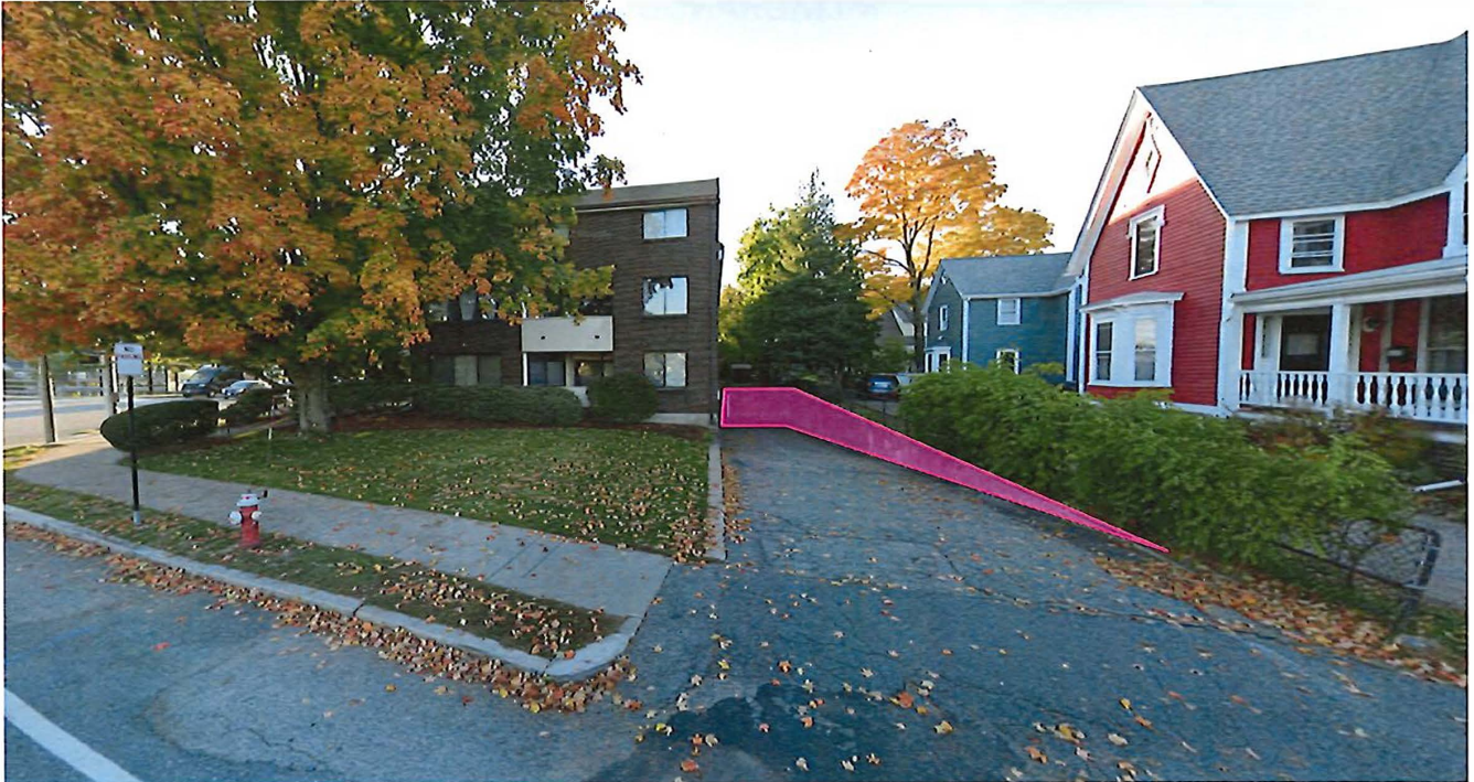
Fully below grade driveway and retaining wall leads to parking beneath the building
