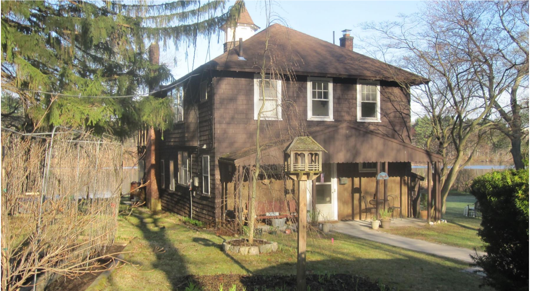
Existing house- street facade
