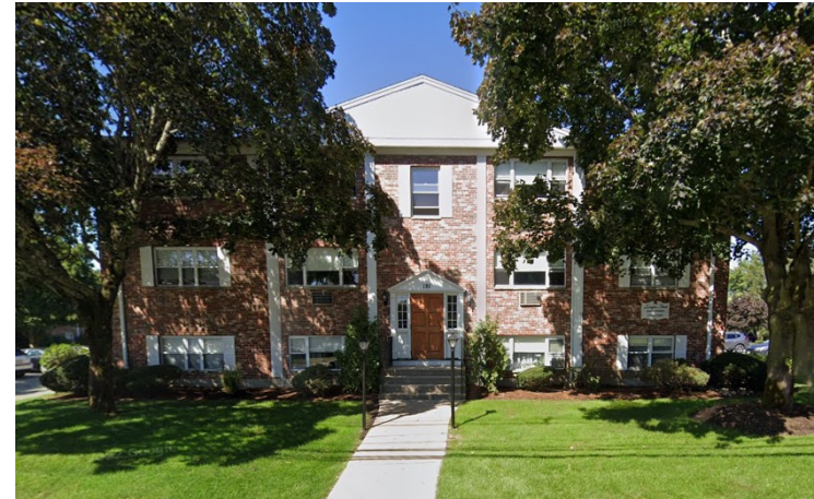
181 LEXINGTON STREET WITH BOILER ROOM
