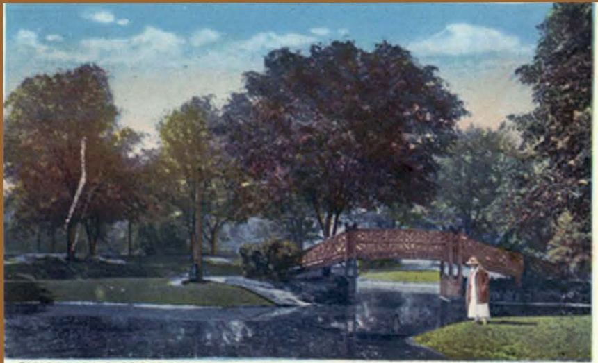
FARLOW PARK--RUSTIC BRIDGE NEWTON MASS
