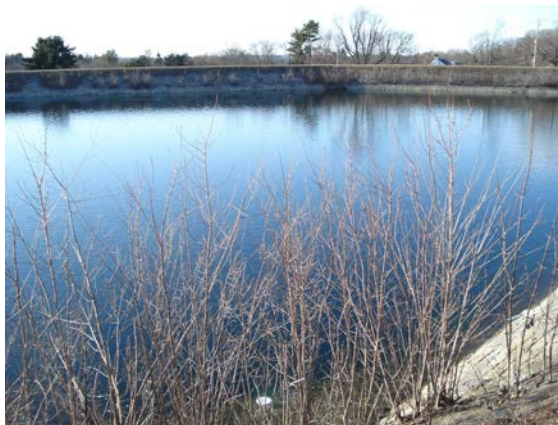
Figure 57: Waban Hill Reservoir. ( Left ) View from berm at southeast corner (Ward/Manet) down to Commonwealth Avenue. ( Right ) View on southern edge of impoundment. Note the trees in the riprap that need to be cut, as indicated in the 2012 MWRA report.
