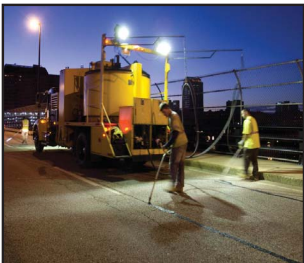
Crack Seal
