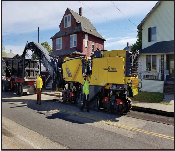
Mill and Overlay
