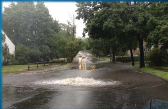
Drain Manhole Overflowing at Dedham Street
