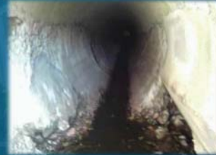
Culvert at Runaway Brook at Grove Street
