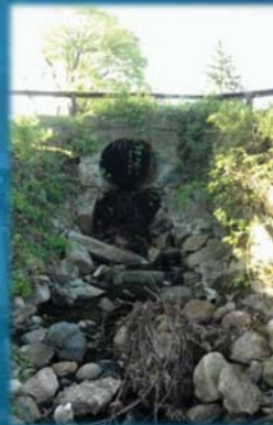
Culvert at Runaway Brook Near Grove Street
