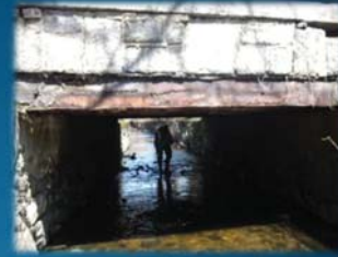
Culvert at Cheesecake Brook at Parsons Street
