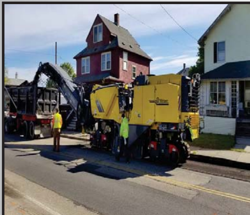
Mill and Overlay
