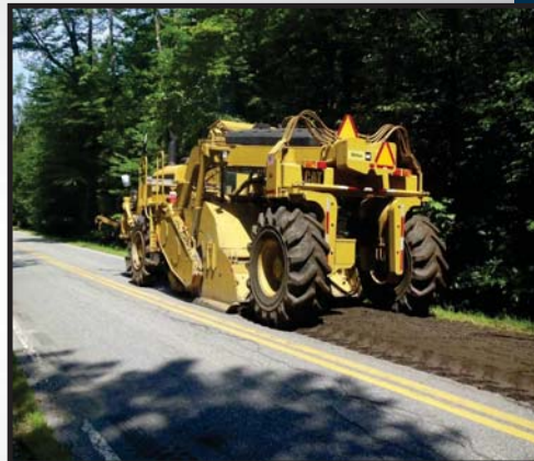
Full Depth Reclamation
