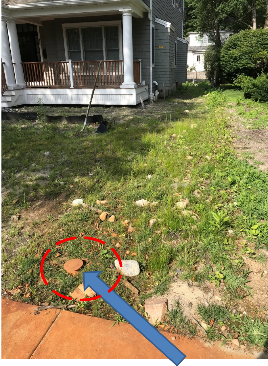
Diffuser discharges to lawn & overflows to sidewalk and street.
