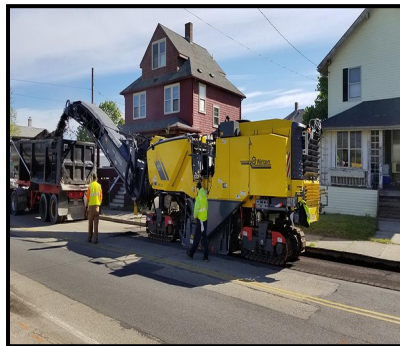
Mill and Overlay
