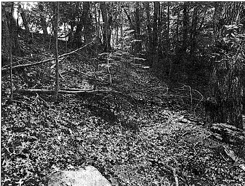
Photo No. 6: Downstream slope from left of the spillway looking left.
