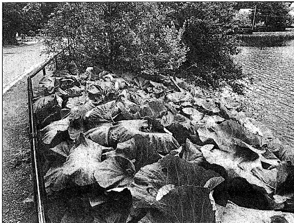
Photo No. 2: Upstream slope right of the spillway.
