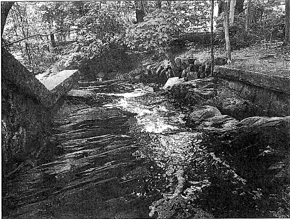
Photo No. 9: Downstream channel at the spillway.
