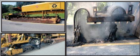
Hot In-Place Recycling
