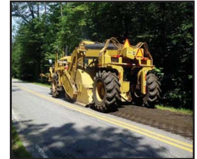
Full Depth Reclamation
