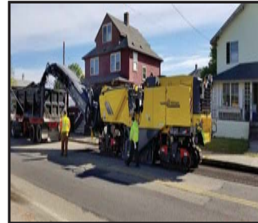
Mill and Overlay
