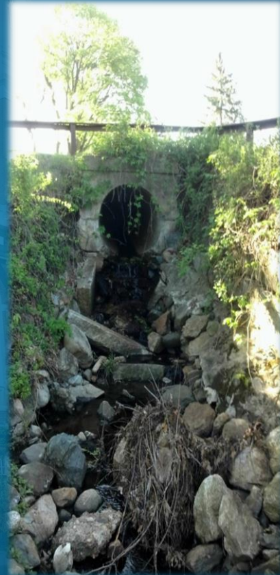
Culvert at Runaway Brook Near Grove Street
