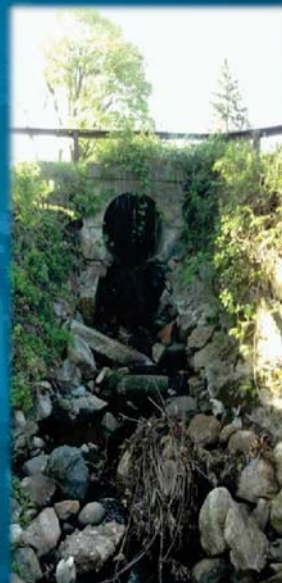
Culvert at Runaway Brook Near Grove Street
