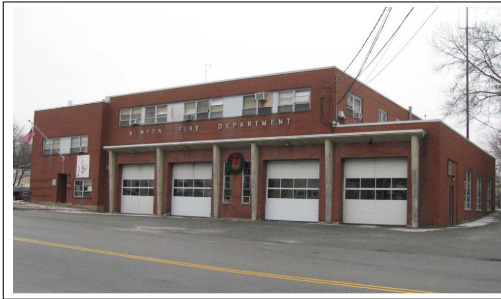
Fire Station #3, 25 Willow Street
