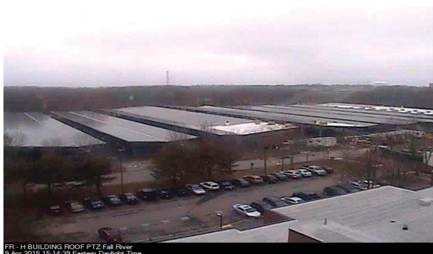
FR - H BUILDING ROOF PTZ Fall River 9 Apr 2015 15:14:39 Eastern Daylight Time
