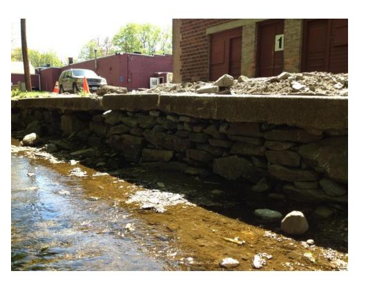
Repaired collapsed rock wall on Cheesecake Brook (Kempton Place)
