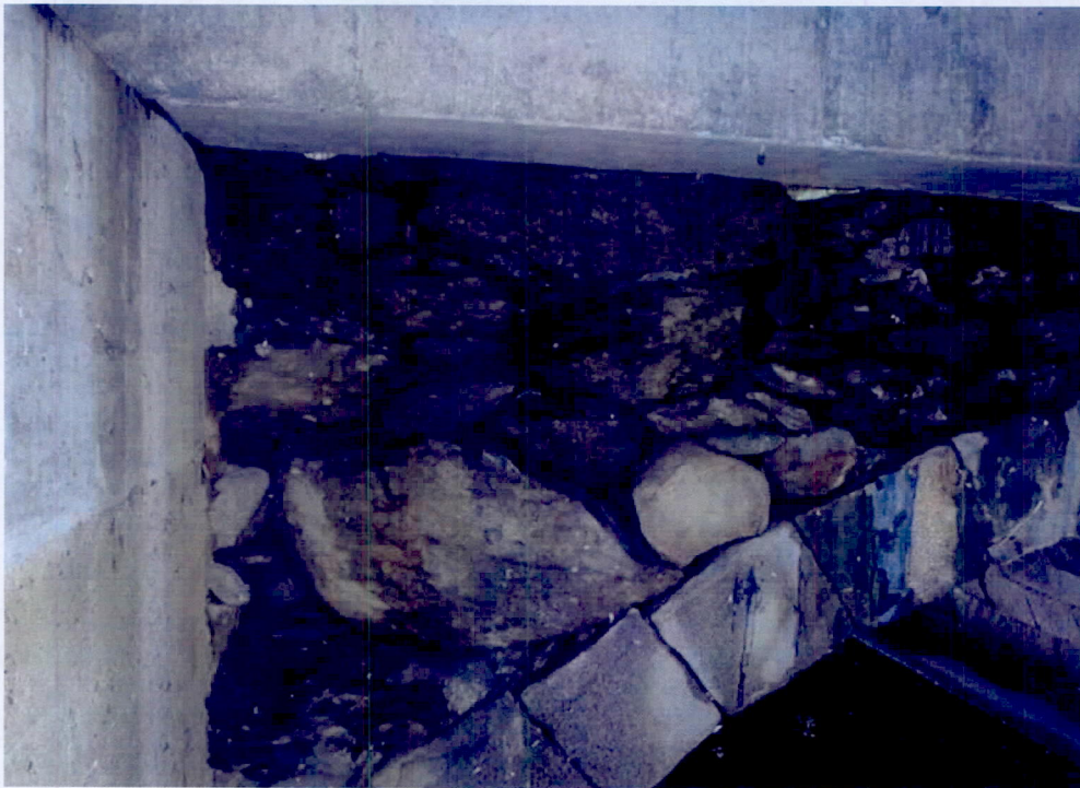
Photo 14: Span 1, north spandrel wall by pier 1.
