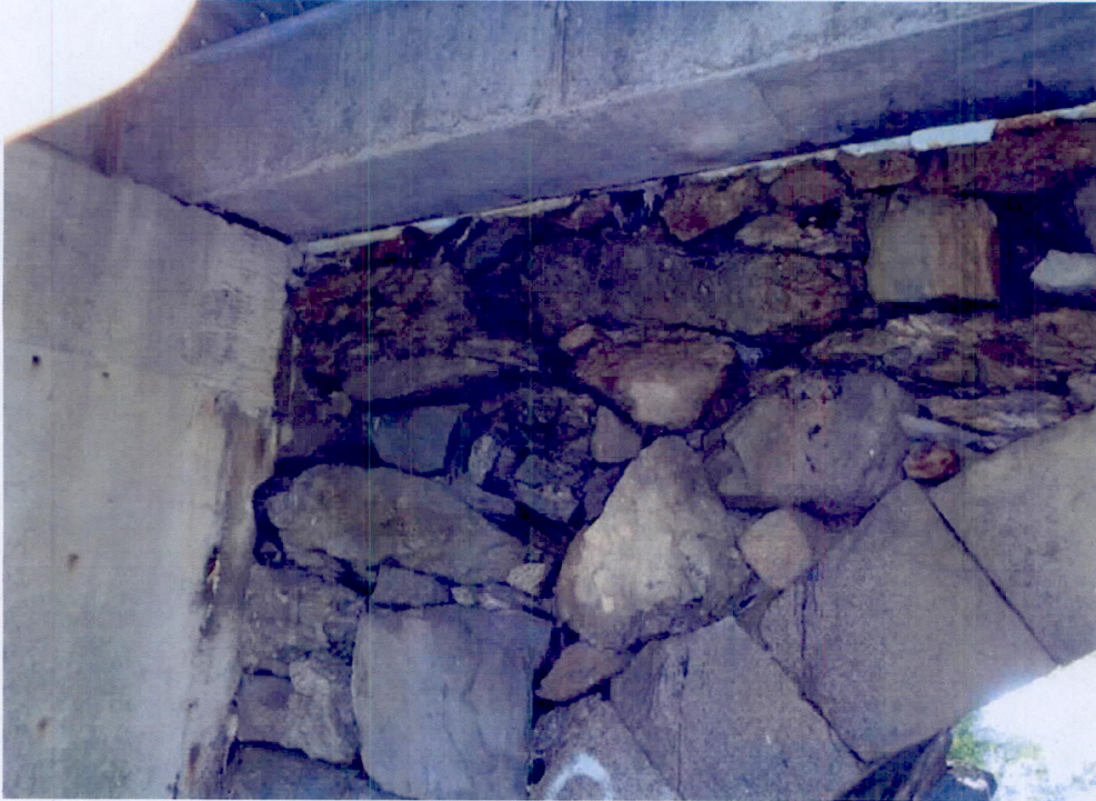
Photo 15: Span 3, north spandrel wall by the east abutment.
