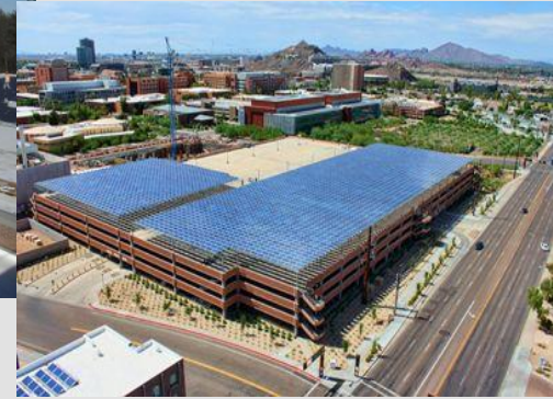
884 kW, Arizona Garage
