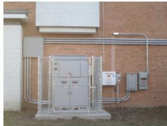
Inverter Installation
