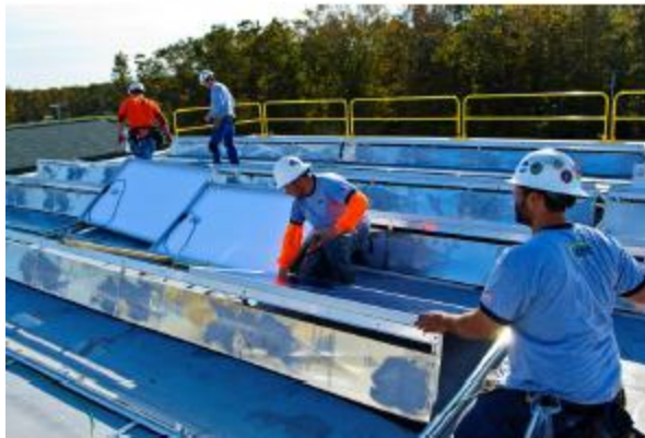
Panel Assembly & Wiring
