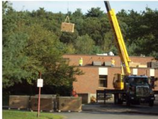
Mobilization & Crane Ops
