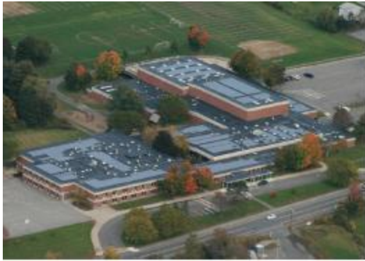
Newburyport, MA: 502 kW 2 Schools and DPW Bldg.
