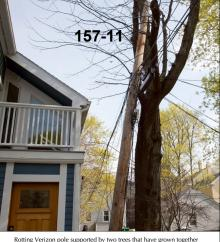
routing verizon pour supported by two trees that have grown together (one of which is also rotting). Note cables going to neighboring homes in 3 directions. We have not been able to use our front door for nearly 4 years because the entry way (steps and patio) could not be built until Verizon finalized the plans for burying the cables.
