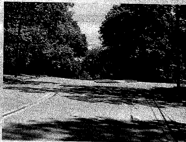
2. Mill St. Facing East at Cedar St.
