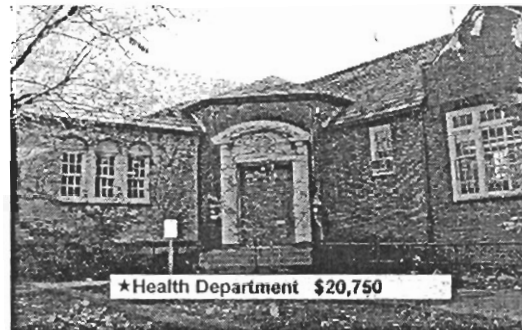
Public Buildings Department FY07
