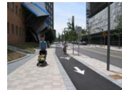
Combined Bike Lane & Walkway
