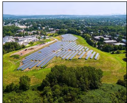
Renewable Energy: Solar array at Rumford Avenue
