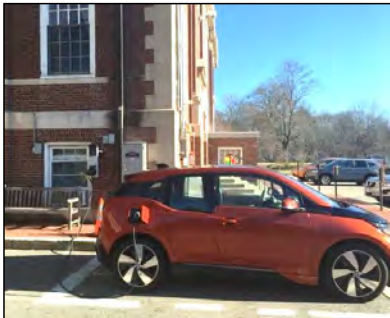
Clean vehicles: City Hall EV charging station
