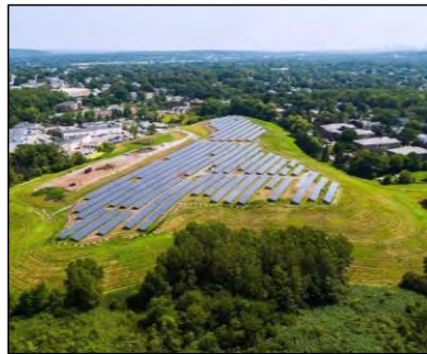
Renewable Energy: Solar array at Rumford Avenue
