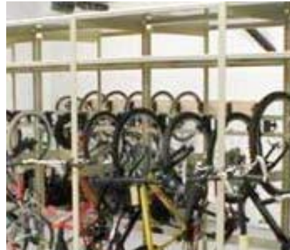
Bike parking & locker rooms
