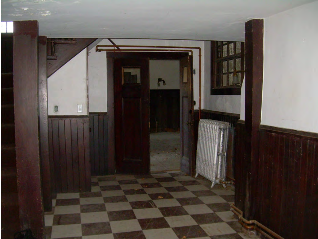
CPC Phase II work: Main Entrance/Lobby (116)
