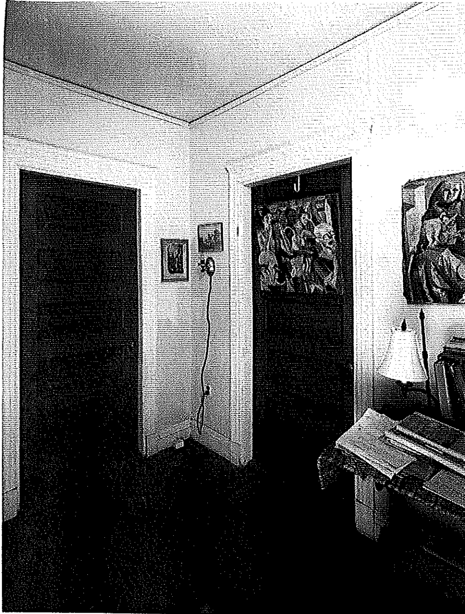
Exhibit B - MA: Newton, 7 Norman Road, PEABODY-WILLIAMS HOUSE Second Story West Hall: Looking Southeast (neg. #54424-A)
