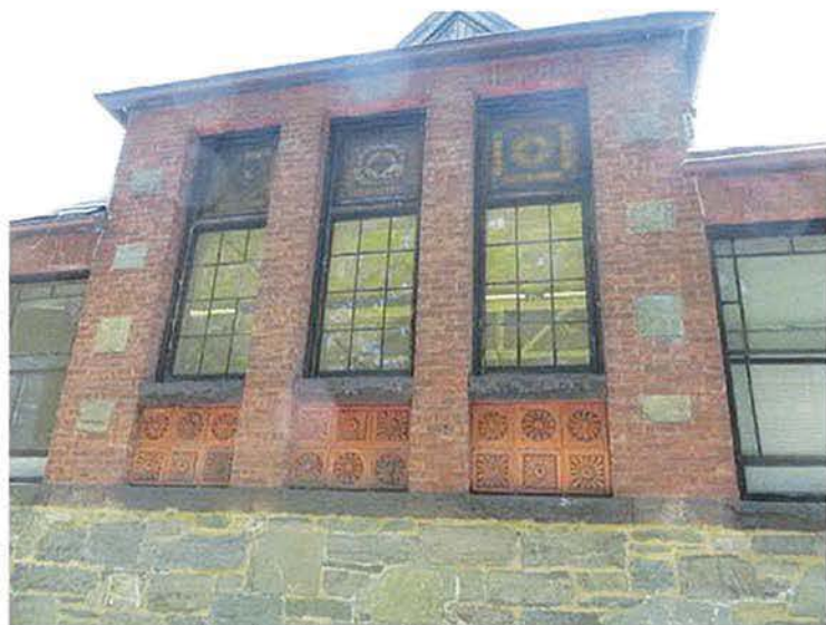
Figure 2: Exterior of ELVAS studio architectural detail
