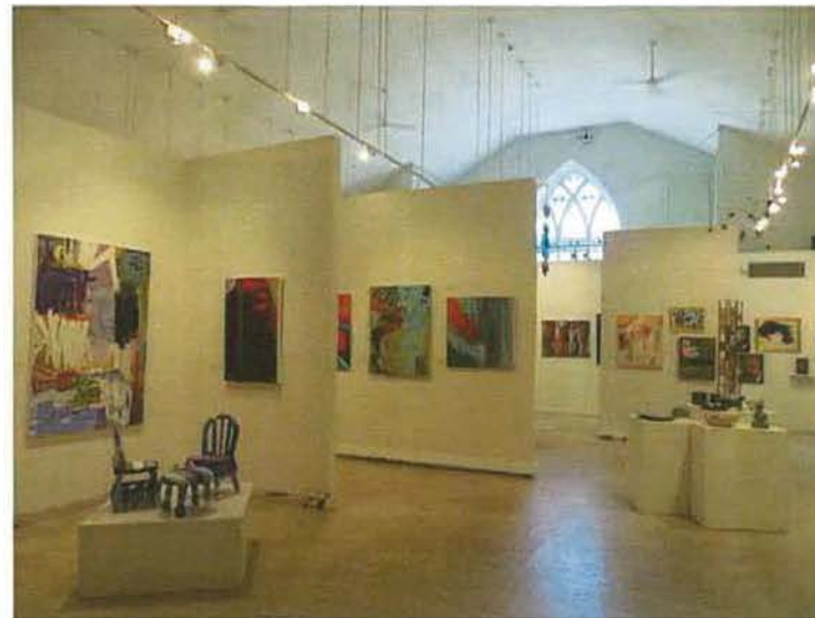
Figure 5: Main Gallery interior, floors in need of repair
