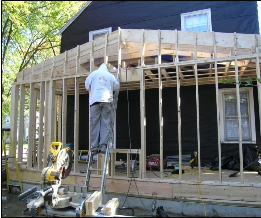
Constructing an accessible bedroom and bathroom for an elderly Newton resident
