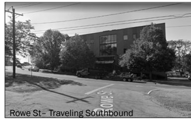
Rowe St- Traveling Southbound
