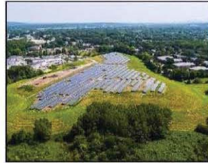
Renewable Energy: Solar array at Rumford Avenue
