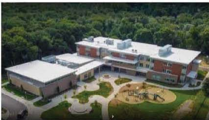
Green Buildings: Zervas Elementary School
