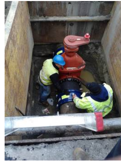
Water system maintenance
