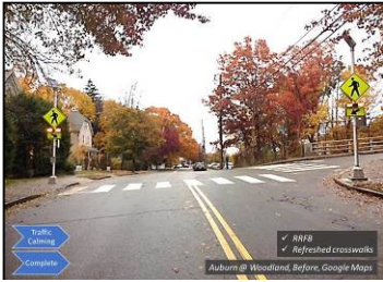
Rapid Flashing Beacons, Auburndale
