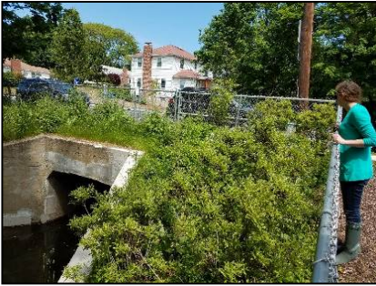
Culvert repairs in Stormwater Program
