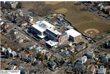
Cabot School Progress 3/20/19
