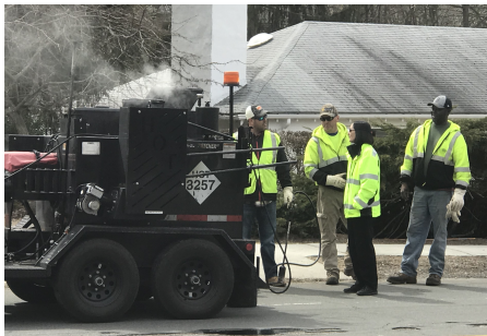
Mayor checking in with Spring pothole filling crew
