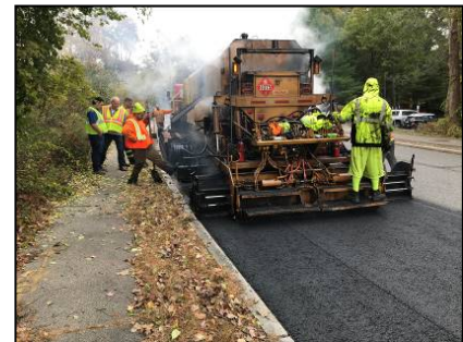
Using Hot in Place asphalt recycling technology
