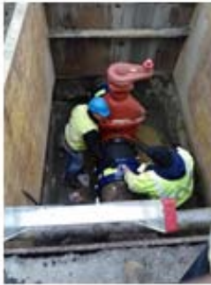
Water Valve Replacement
