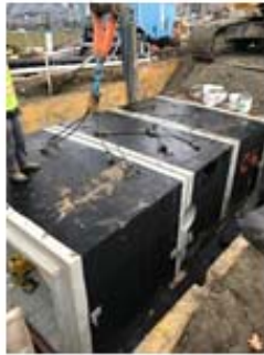
Box Culvert Installed for Laundry Brook at Cabot School
