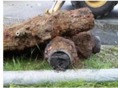
Replacing Tuberculated old water mains
